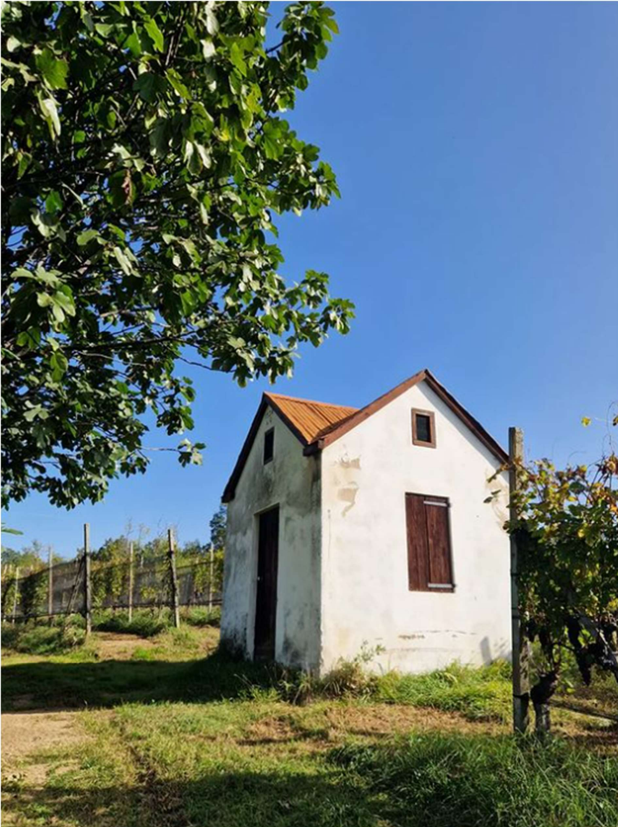
A farmer's shed in the middle of Cavazucchi parcel in Bramaterra .
